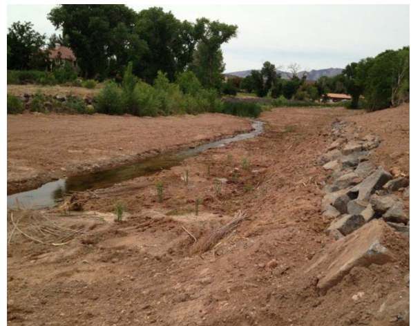
Toe rock and bioengineering (pole plantings and brush layers) near the Monterey Subdivision and Sunbrook Golf Course in St. George, UT. Funded through DR-1955 HMGP. Image credit: FEMA.
