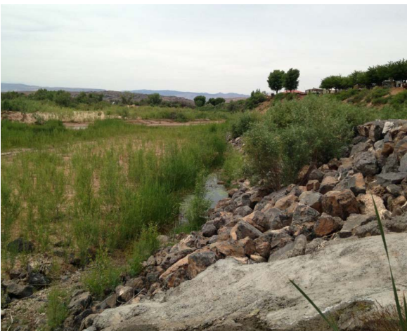
Bank Stabilization Project to protect critical public infrastructure - the Millcreek Electric Generation . Image credit: FEMA.
