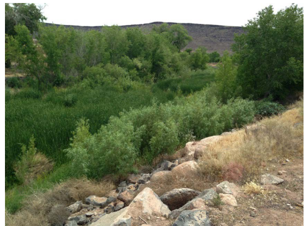
Erosion protection improvements on the Santa Clara River. This project used bioengineering (pole plantings) to supplement riprap and is a good example of the city's overall vision. Image credit: FEMA.
