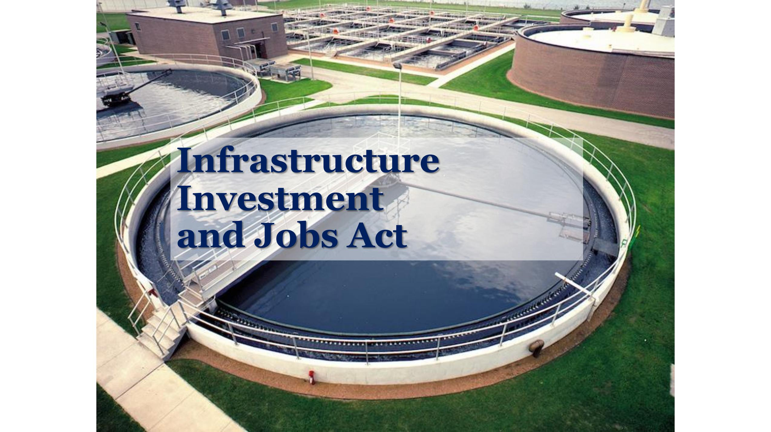
An aerial photograph of a modern wastewater treatment plant. The facility features several large, circular clarifiers with metal railings and walkways. In the background, there are rectangular aeration basins with a grid of pipes and walkways. A brick building is visible on the left side of the plant. The entire facility is surrounded by green grass and paved walkways.
