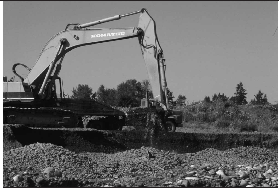
Gravel mining on the Willamette River, Oregon
