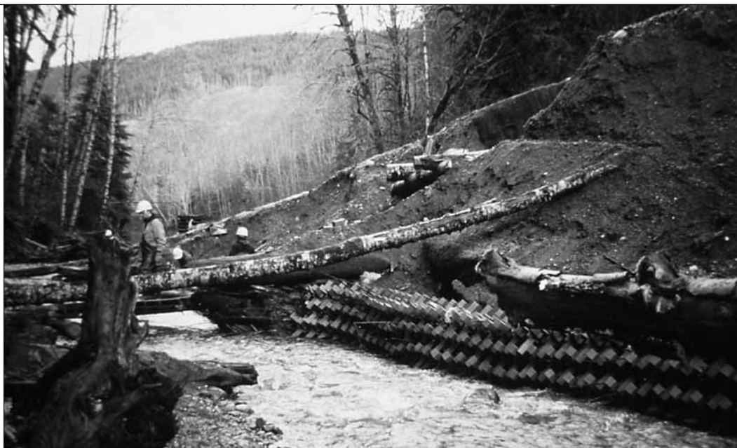
A-jacks are installed on the Upper Skagit River in Washington to control erosion.
