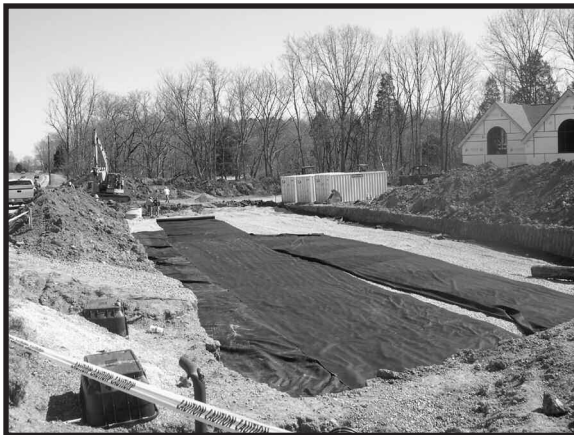
The County used underground detention and pervious concrete in the construction of the parking lot for Powell Branch Library.
