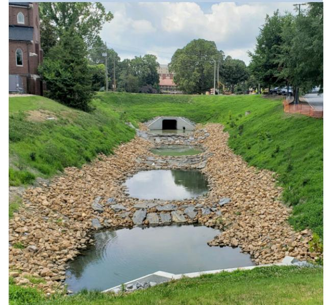
*A regenerative stormwater conveyance system in Greenville, NC. Photo courtesy of WK Dickson & Co., Inc.*
